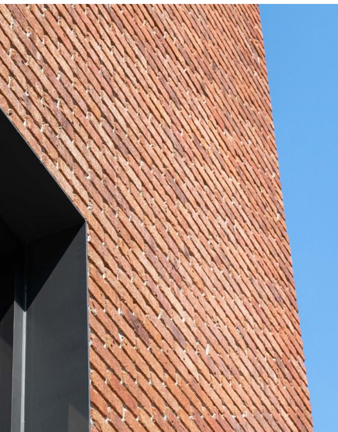
A wall panel with a thin-brick face. Photo: Clark Pacific.
