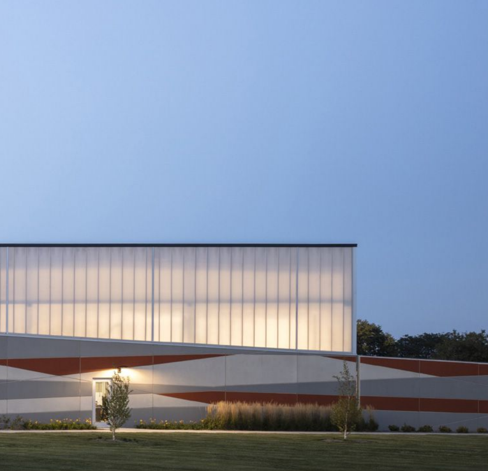
The precast concrete panels decrease in size as they run along the front of the building. Photo: AJ Brown Imaging.
