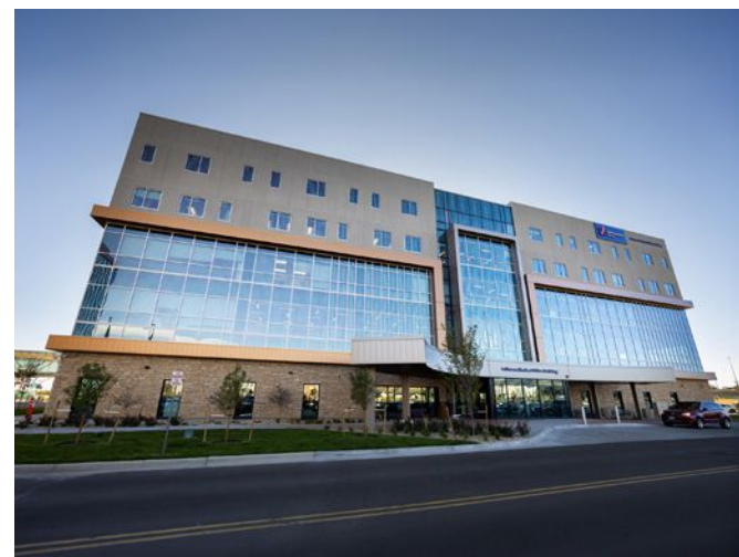
Intermountain Health Lutheran Medical Office Building, Wheat Ridge, CO. Wells provided design-assist services to convert the building envelope to a unitized façade system.
