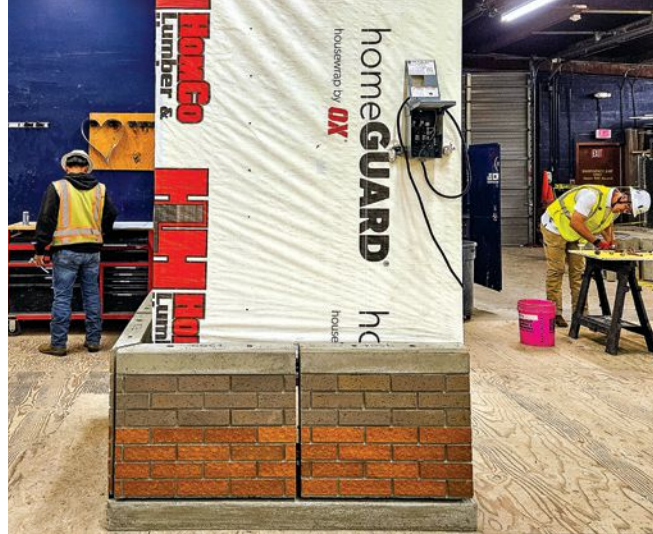
Four of the eight miniaturized precast/prestressed concrete panels are installed on a team’s final projects in the CM lab.
