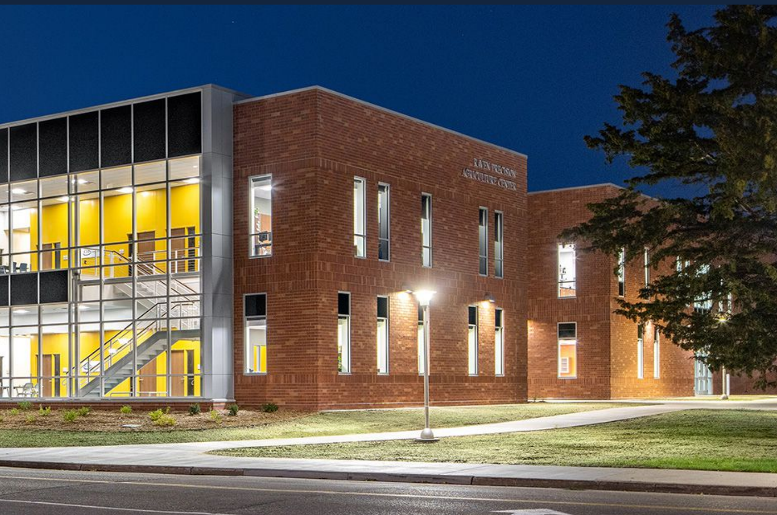
Precast concrete walls made the south side of the Raven Precision Agriculture Center possible, enabling the construction of the high- and mid-bay spaces needed to house large agricultural equipment. Photo: Jordan Powers Photography.
