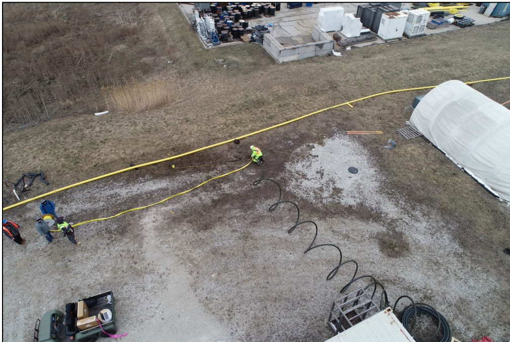
Figure 5. Overhead view of Boretrace™ tracer wire installation
