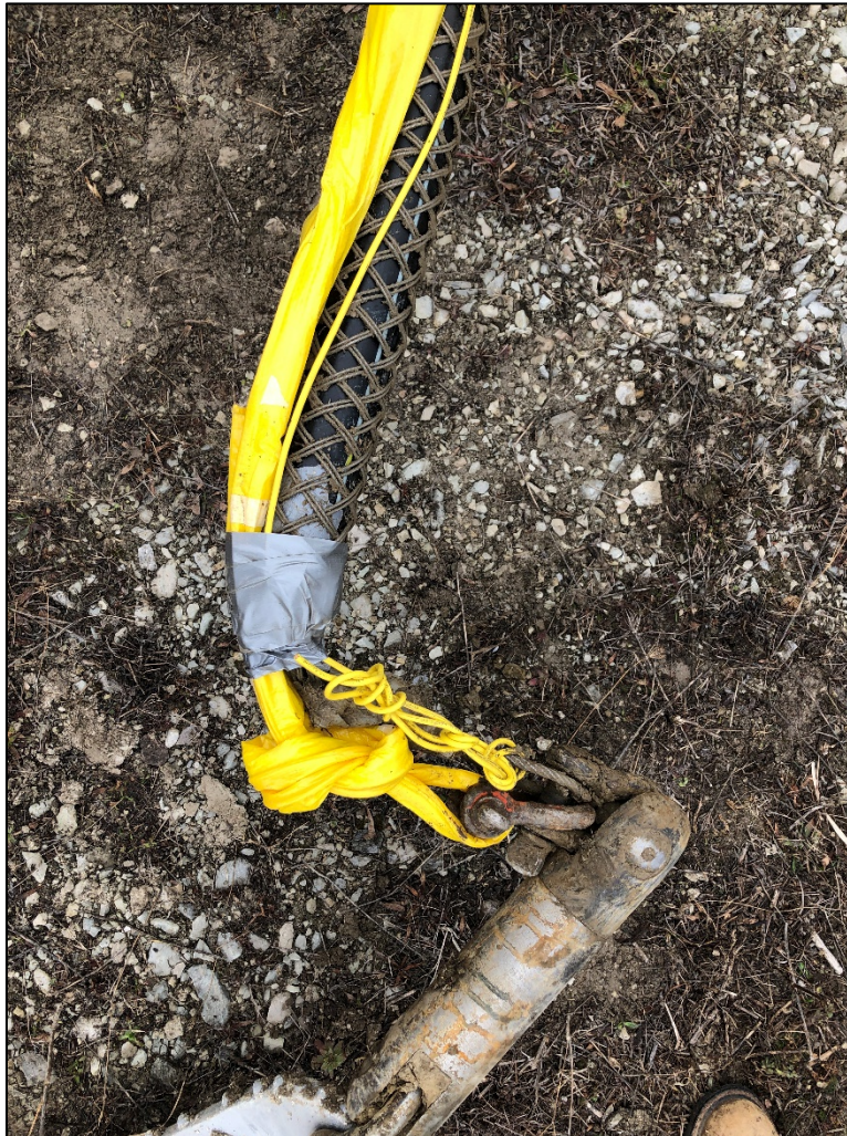
Figure 3. Installation attachment of tracer wire products
