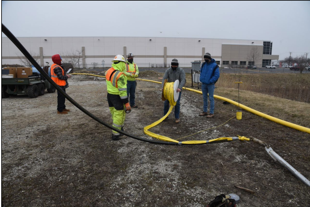
Figure 4. HDD Installation with Boretrace™ tracer wire
