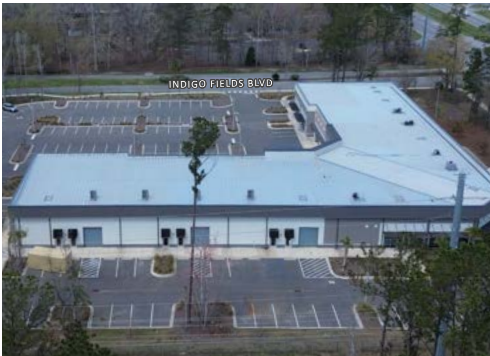
ROLL-UP DOORS ON SOME SUITES
