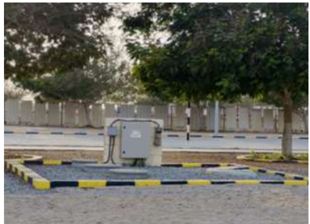
On-site sewage treatment plant installed at BDC facility
