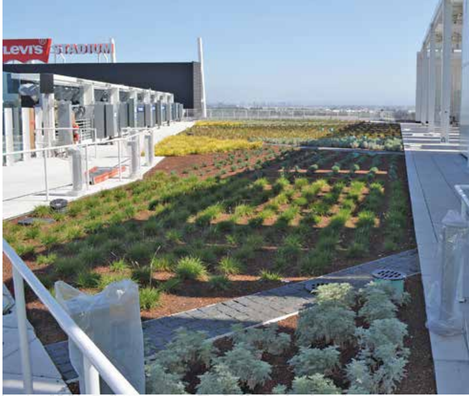
The green roof on the Suite Tower uses a variety of shallow root, hearty plants that require minimal maintenance. It is part of the stadium's sustainable design to keep the building thermal envelope cooler.
