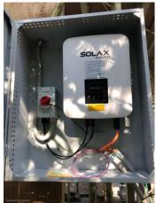
2. Inside the inverter enclosure, you'll find the DC isolator switch. Simply cut the cable tie and turn the switch on.
