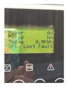
Grid Loss Fault: This typically means that something is not switched on. Complete the shutdown procedure that is labelled on the inverter and then re-complete these steps.
