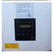
3. The inverter will start up, and the screen will say "checking". After a few seconds, it will then countdown from 120. After the countdown, the inverter will show "normal", and the PAC number will rise. This is the solar's current production.
