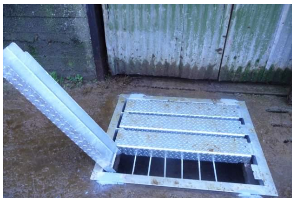
Slurry mixing point
