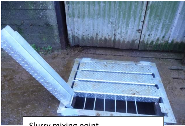
Slurry mixing point
