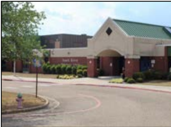
Image 1: South River Elementary School
