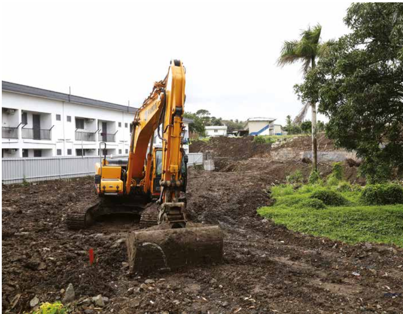
Road construction in Suva
