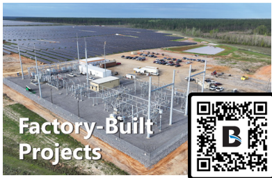
Agile EPC of a 138/34.5kV substation for a 125MW solar farm in Louisiana
