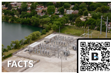
EPC of a flexible AC transmission system (FACTS) involving two 300 MVAR 138/15kV static VAR compensators in Illinois
