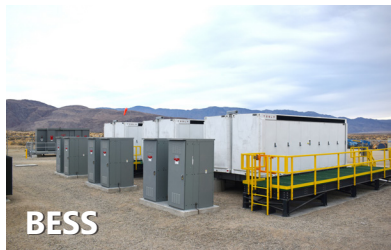
EPC of a 7.3MW/14.6MWh battery energy storage system (BESS) in California
