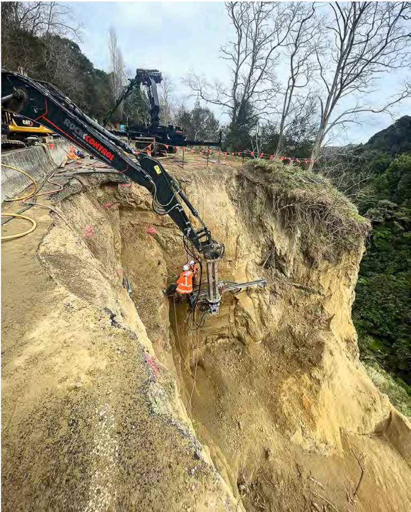
Drilling works underway at the Otoko site. For this work, heavy machinery is positioned on the road and is being used to access hard to reach areas and drill metal bars into the base beneath the road.
