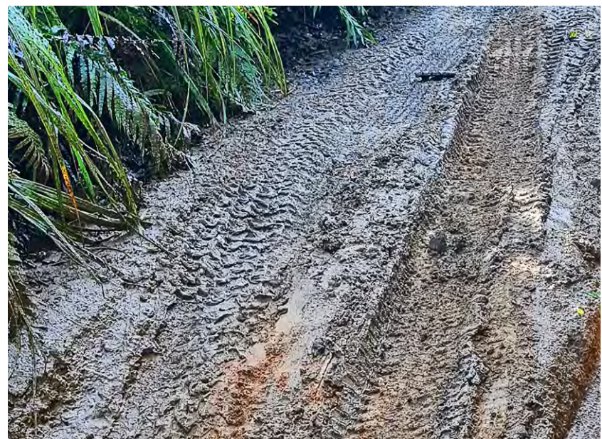
Four-wheel drive vehicles cause damage to the T42 in winter conditions. Photo: DOC.
