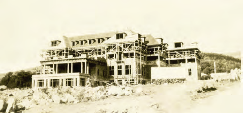
Chateau Tongariro under construction, 1929. Almost 100 years on, the future of the iconic building is still not sorted.
