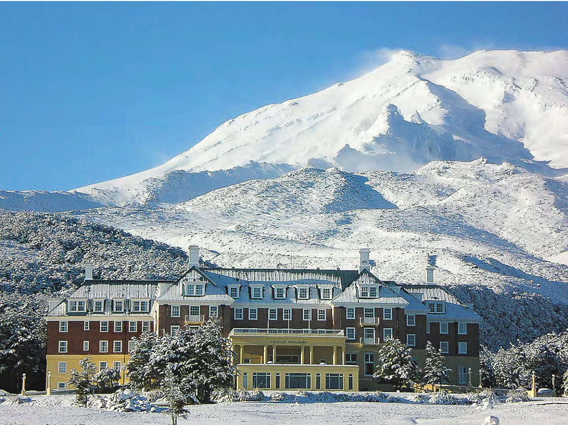
Ruapehu’s mayor Weston Kirton is welcoming Government’s proposed changes to earthquake-prone building rules, which could be a game-changer for restoring the Chateau Tongariro – closed since February 2023 partly due to seismic safety concerns. Photo: Maree Surrey.
