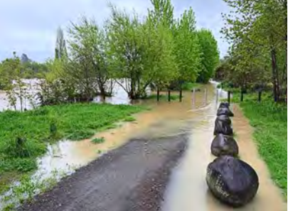
The Whanganui river breached its banks, flooding the river walkway.
