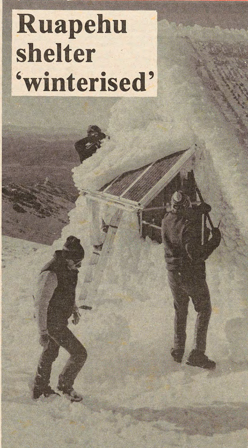
On a perfect sparkling day near Mt Ruapehu's crater lake recently solar panels on Dome Shelter were lowered for the winter. MWD radio technician Barry Hishman, and park assistant Simon Gardner de-ice the panels with park ranger Paul Dale in the foreground. Through the winter ice builds up to twice the seven-metre length of the shelter and three metres on top.
