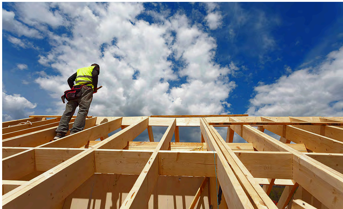
Council's new Datascape building consenting system will allow applicants to track the progress of their building consents online, receive automatic notifications when updates occur, and interact with the building team through a modern end-to-end digital system.
