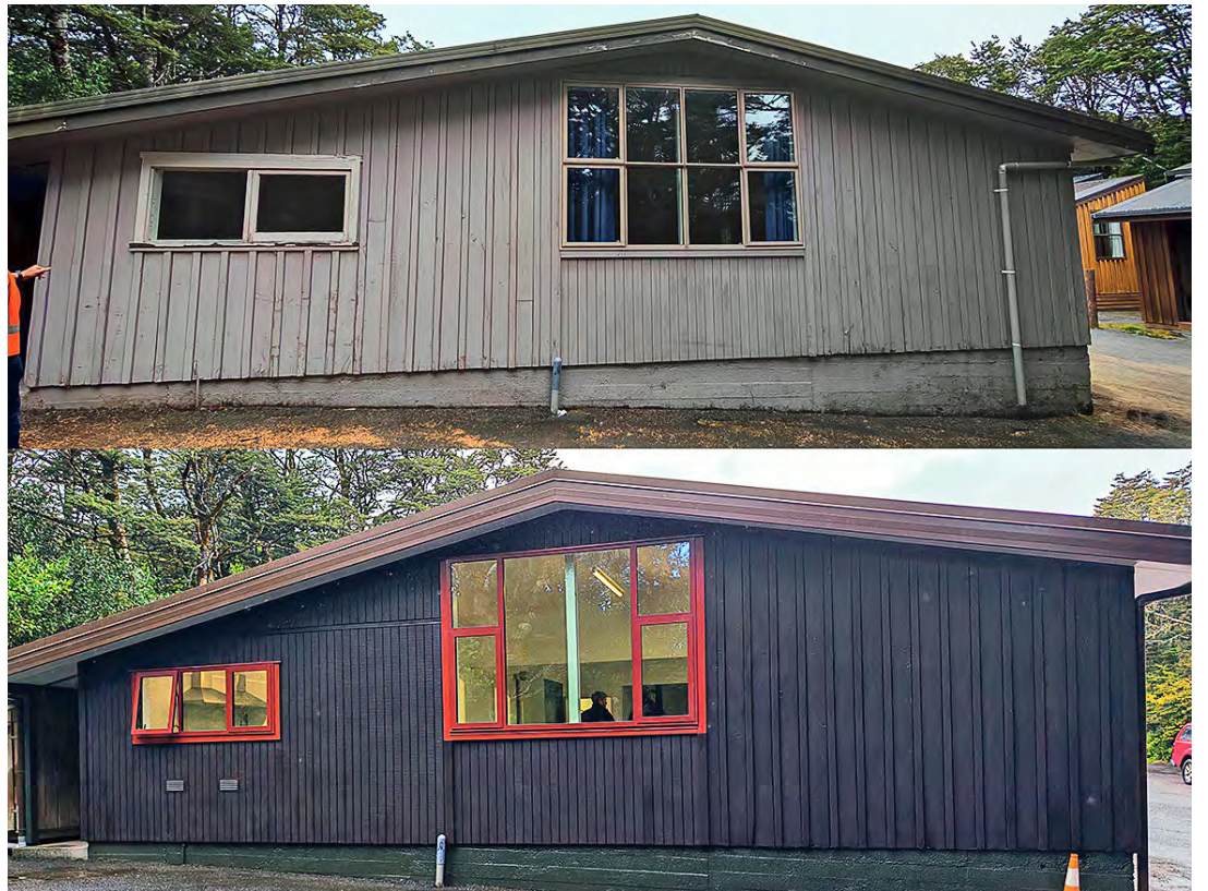
Exterior reno, before and after: a lick of paint and some fresh glazing. Photo: Citycare Property.
