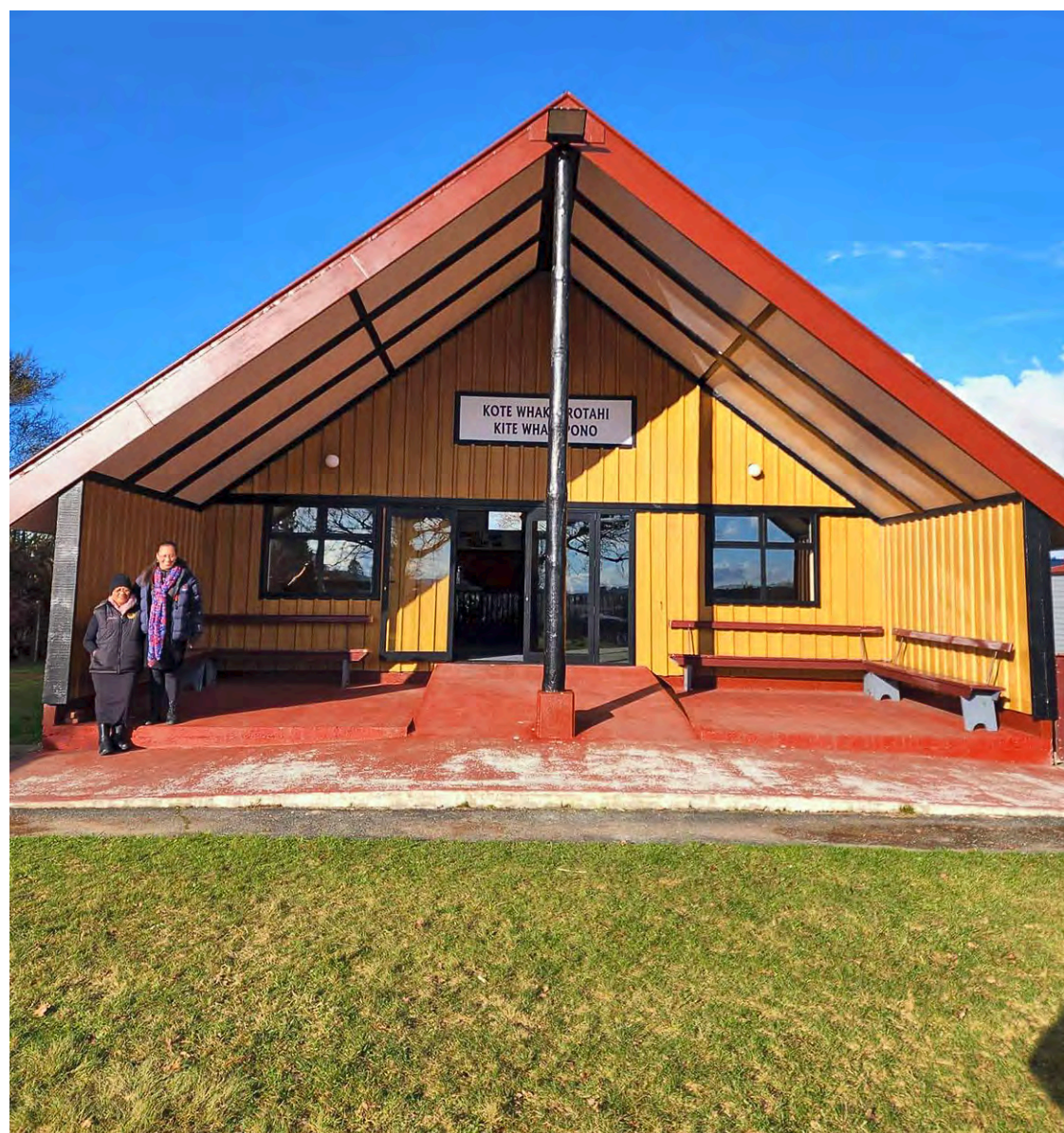
Raetihi Marae will not be available for functions until the New Year, but the Trust promises a much-improved facility once work is complete. Photo: Raetihi Marae Trust.
