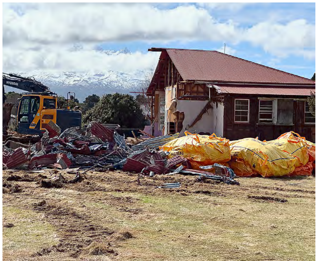
Rangataua School is no more, with the last of the structure knocked over on Wednesday 27 August.
