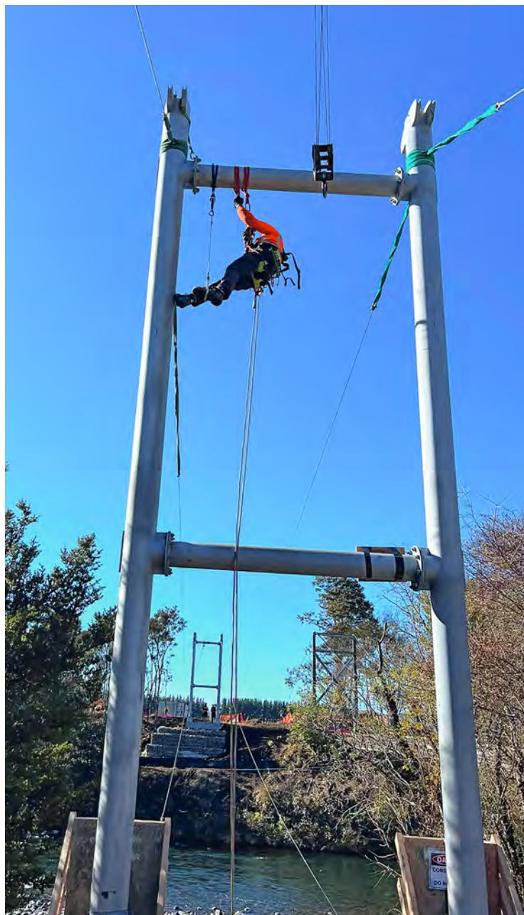
Climber Jeremy Hamer working at height on a swing bridge. Photo supplied.
