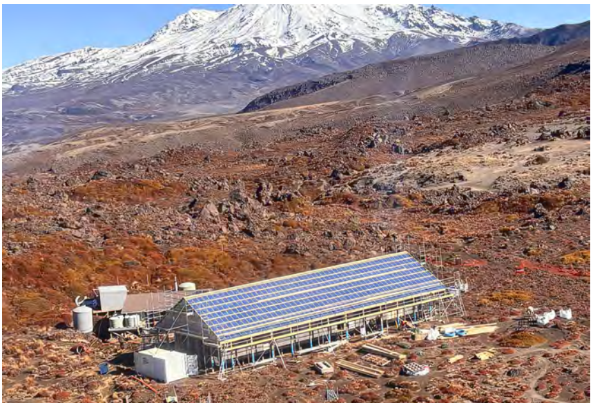
The new Oturere Hut – opening delayed until December. Photo: DOC.
