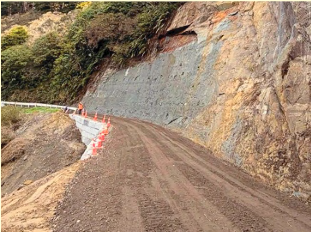
Ruatiti Road repair has now received engineering sign-off and approval and the road is now open, reports RDC. There are some minor works still to be completed, which will be undertaken under normal traffic management rather than requiring a road closure. RDC urges drivers to continue to drive with care through the work area. Photo: RDC.
