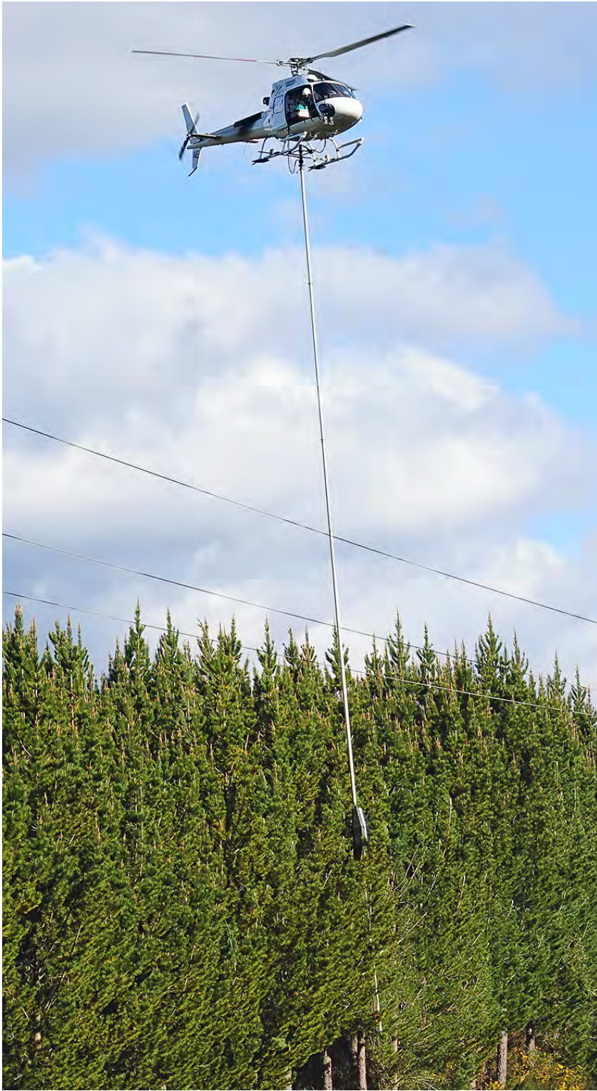
The helisaw in operation alongside TLC's live 33kV Kuratau power line in Rotoaira Forest, where vegetation was safely cleared without turning power off to customers.
