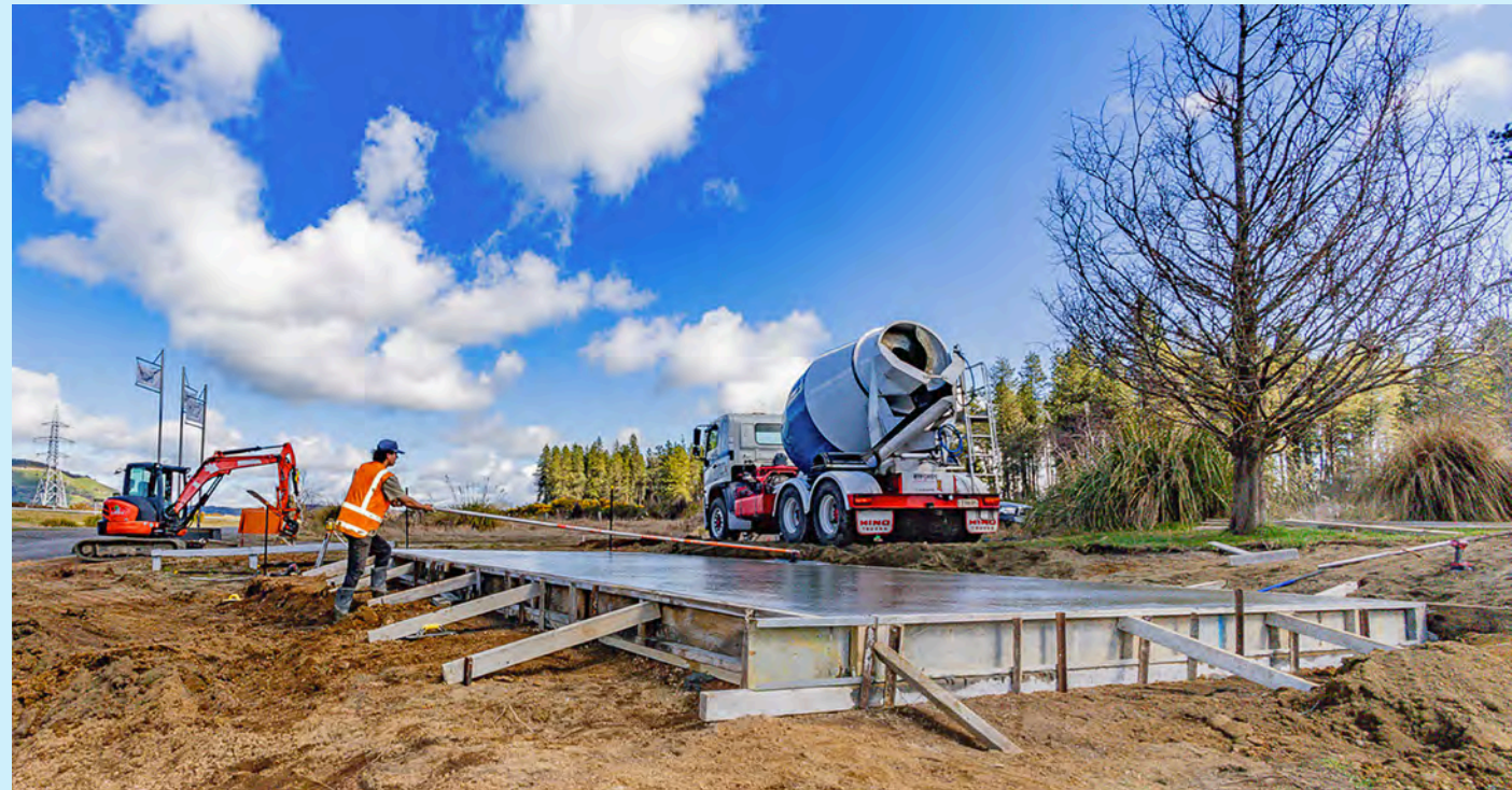
Anton Fraser from RFL puts the finishing touches on the concrete slab for the new shelter for visitors to the Tangiwai Rail Disaster Memorial – part of a $150,000 project to upgrade the memorial site, led by Ruapehu Lions. The shelter is to be in honour of the families and others affected by the 1953 rail disaster that saw 151 people lose their lives. The shelter will also feature a deck where people can sit and view the memorial site and the river, towards Mt Ruapehu. There will be information panels and a path leading from the shelter to the memorial. Project leader Bob Norling said they have so far raised $135,000, some of the money coming from a Pride of Place grant. A 4WD safari next year is also running, with funds to go to the project (see separate story). The project is a joint effort including Ruapehu Lions, Ngāti Rangī and the Ruapehu District Council. Photo: Glyn Hubbard.
