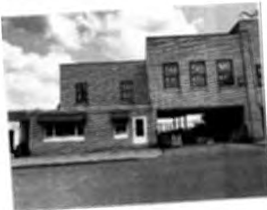
Side of building from Church St. as of 8.11.25
