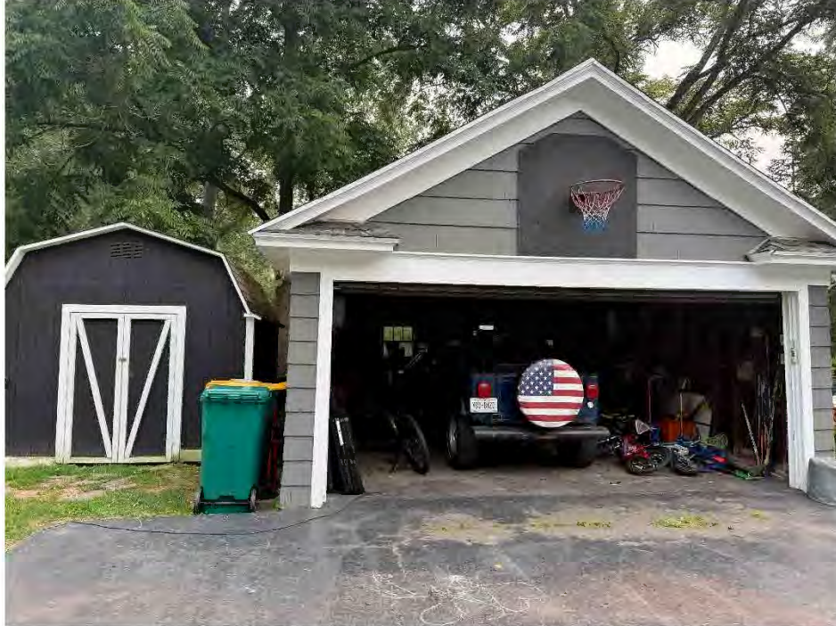
Figure 1 - East facing elevation of existing garage & shed
