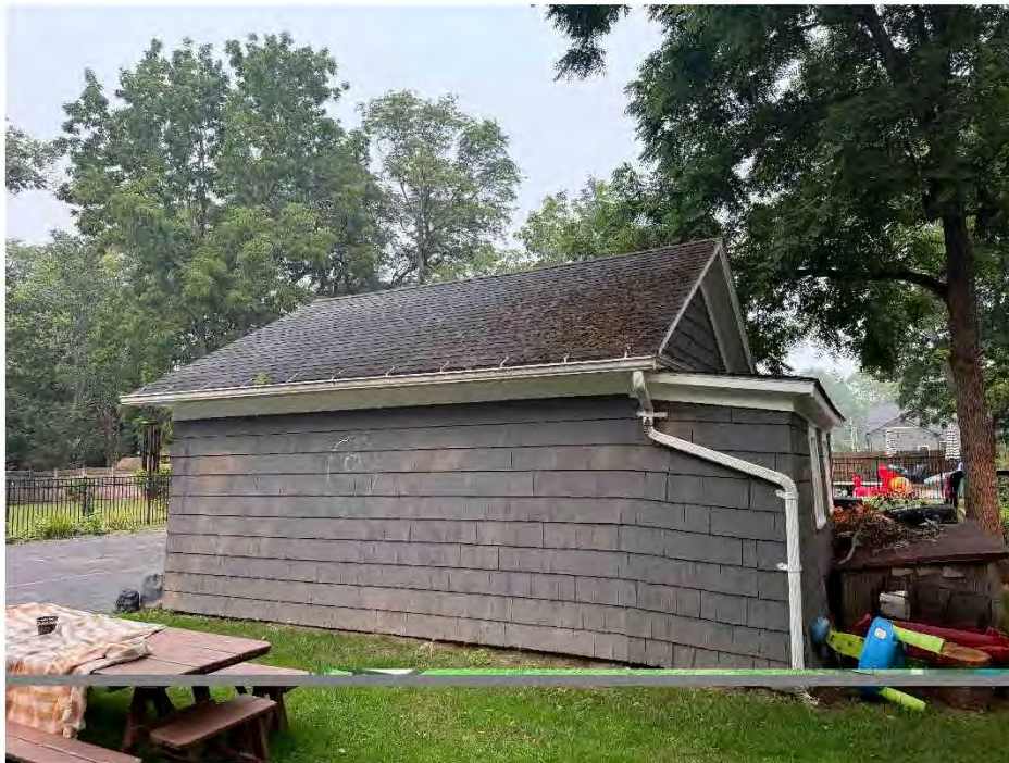
Figure 2 - North facing elevation of existing garage
