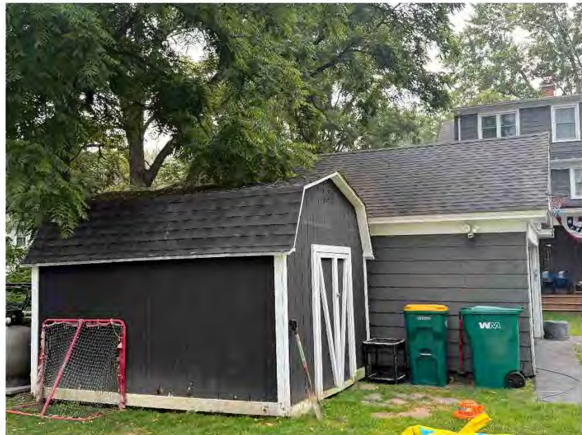
Figure 4 - South facing elevation of existing garage & shed.
