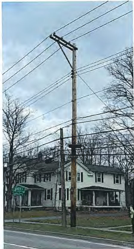
EXISTING POLE PHOTO
