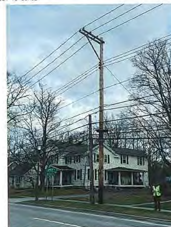
EXISTING POLE PHOTO
