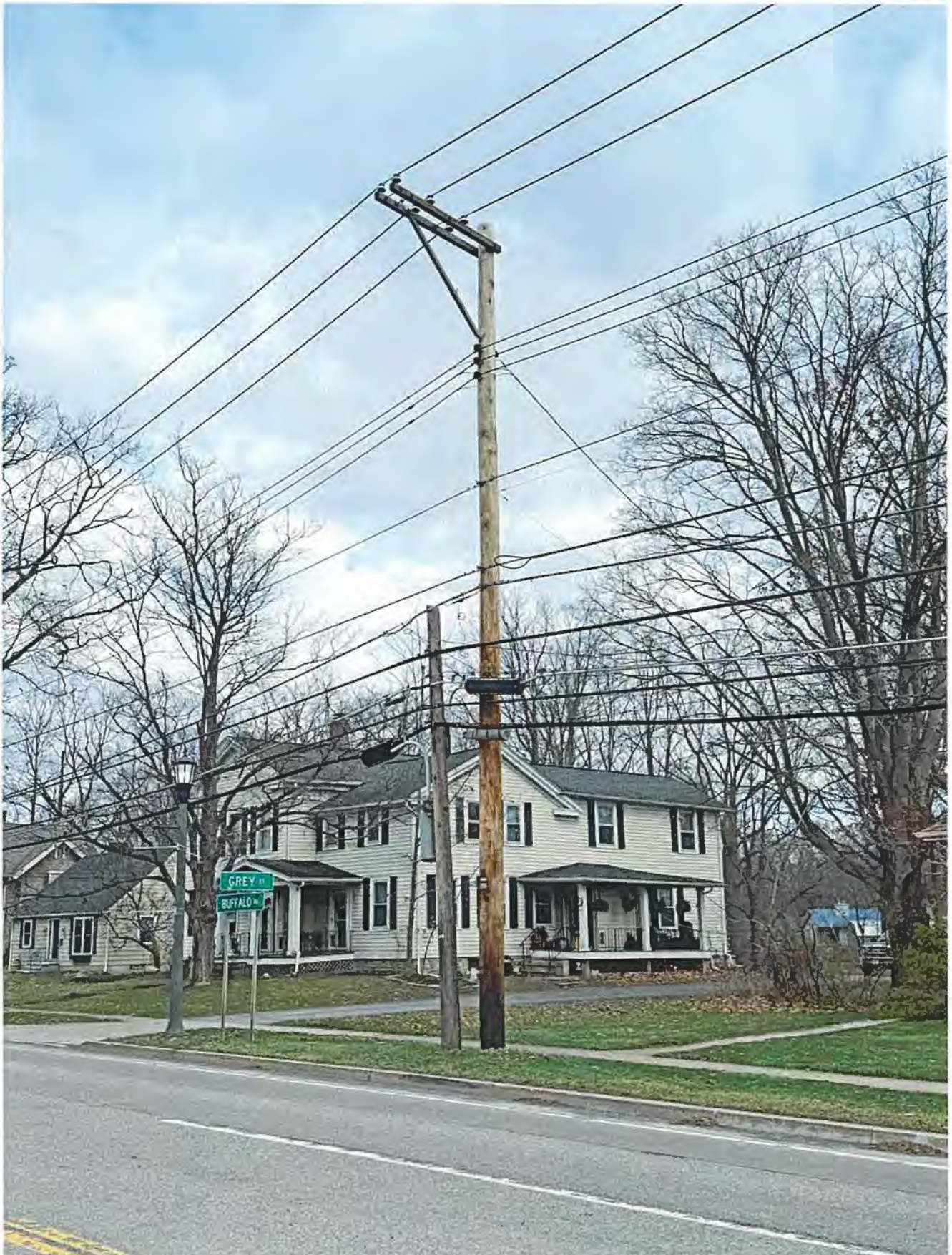
NOVA PARK EXISTING CONDITION LOOKING NORTH
