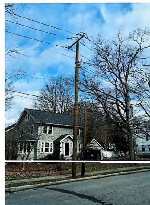
EXISTING POLE PHOTO
