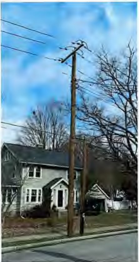
EXISTING POLE PHOTO
