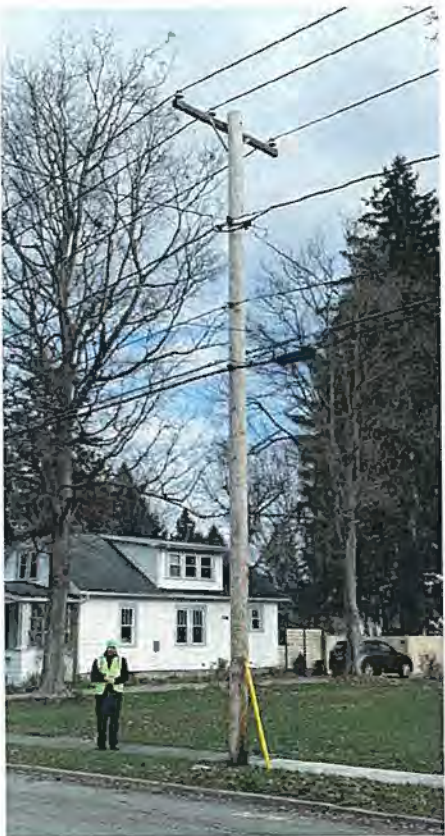
EXISTING POLE PHOTO
