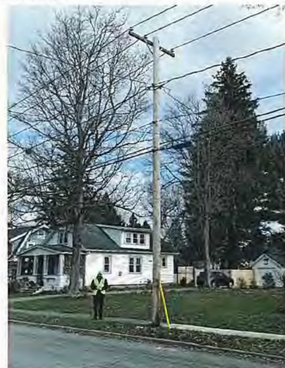
EXISTING POLE PHOTO
