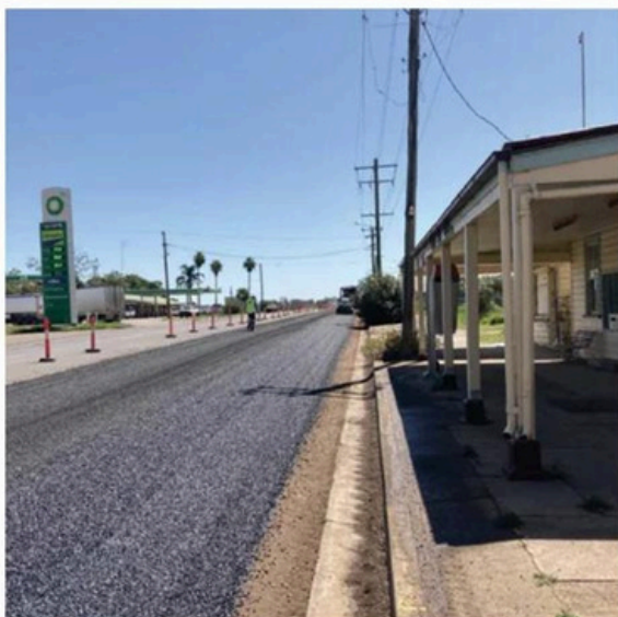
Pavement upgrade on the Newell Highway (image source Transport for NSW)
