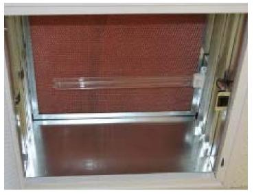
ASIET, Inc. manufactures and distributes 7724-S, an air purification system that improves indoor air quality through UVC light and photocatalytic cell technology rather than filters. The 7724 is a standard, commercial ceiling mount in-duct multi-stage photocatalytic oxidation (PCO) system.
