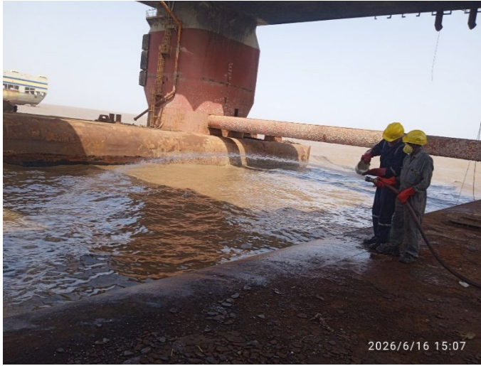
Spraying Oil Spill Dispersant Type III/II for efficiently combating oil spills during high tide
