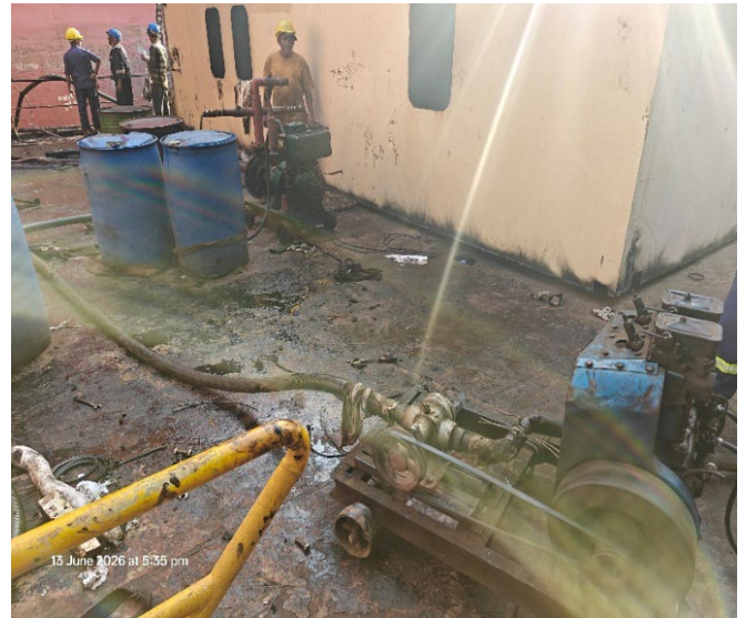
Setting up oil removal pumps and started transferring oil from the pontoon to the barge's empty tanks.
