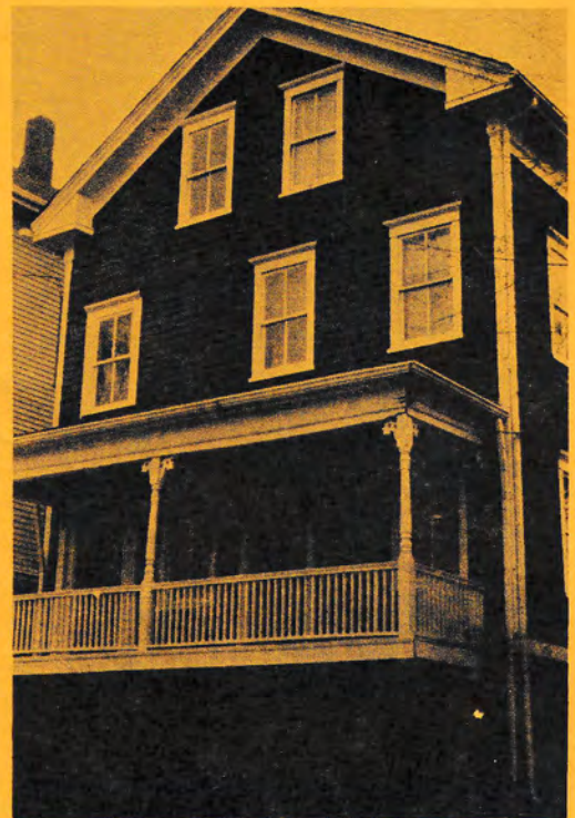
69 Evergreen Street: AFTER
