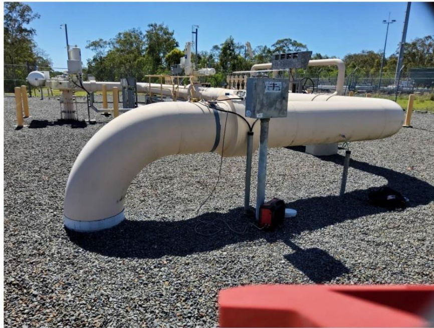
Figure 5. 24NB Gas Riser No.2
