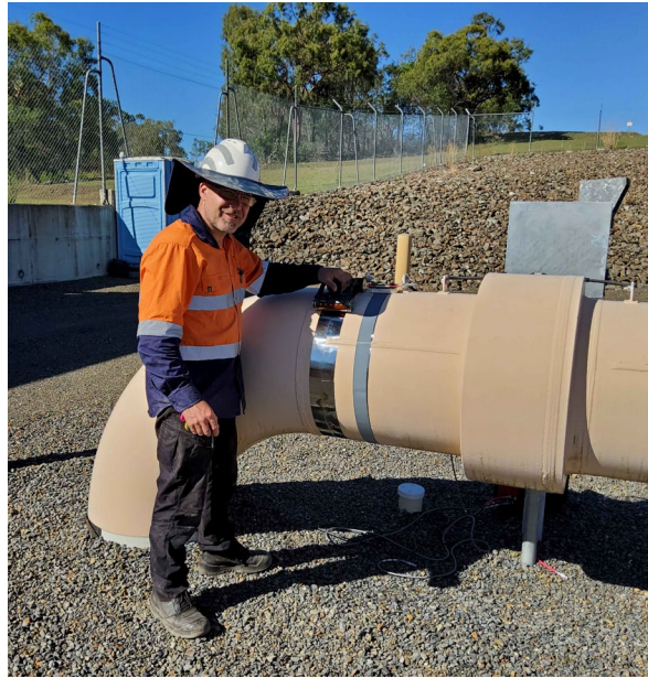
Figure 1. Soil-to-Air Gas Riser Interface
