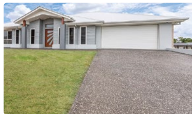
DRIVEWAY Exposed aggregate or plain brushed concrete Type & quantity as per plan/spec
