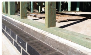
TERMITE MANAGEMENT Termimesh system As per plan/spec
