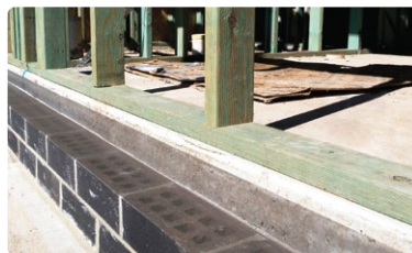
TERMITE MANAGEMENT Termimesh system As per plan/spec
