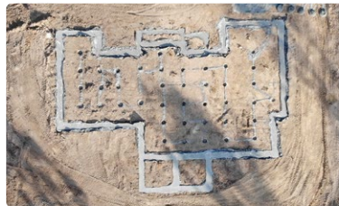
CONVENTIONAL FOOTINGS & SLAB M site with cut/fill to suit* As per plan/spec
