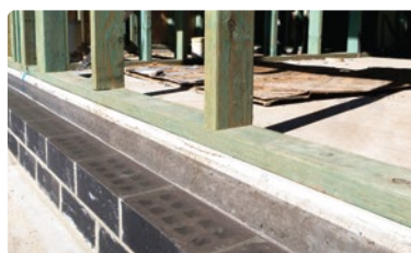
TERMITE MANAGEMENT Termimesh system As per plan/spec
