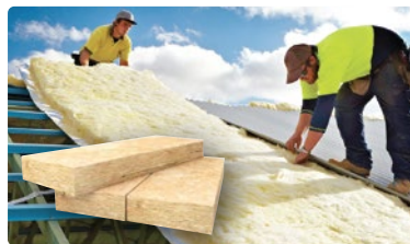
INSULATION R3.0 batts & Anticon blanket As per spec
