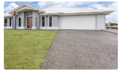
DRIVEWAY Exposed aggregate or plain brushed concrete Type & quantity as per plan/spec
