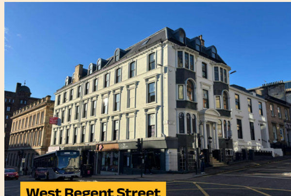
West Regent Street Office
