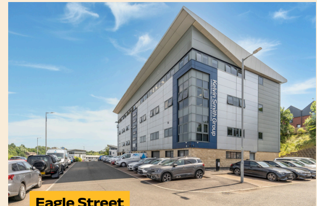
Eagle Street Office
