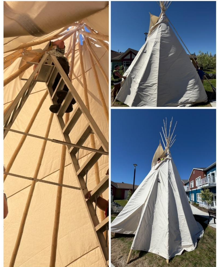
An almost finished 18' teepee project takes shape
