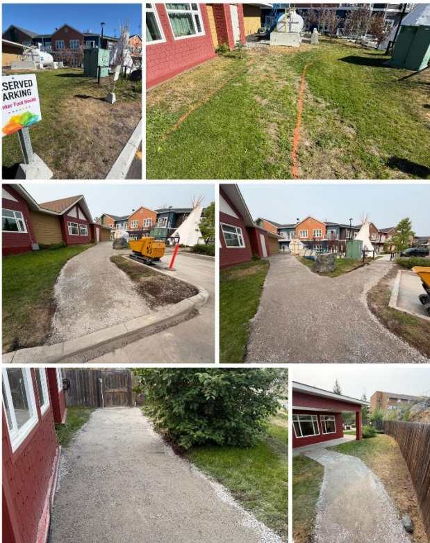
Before and after site preparation
