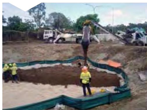
Backfilling over geotextile in a detention basin
