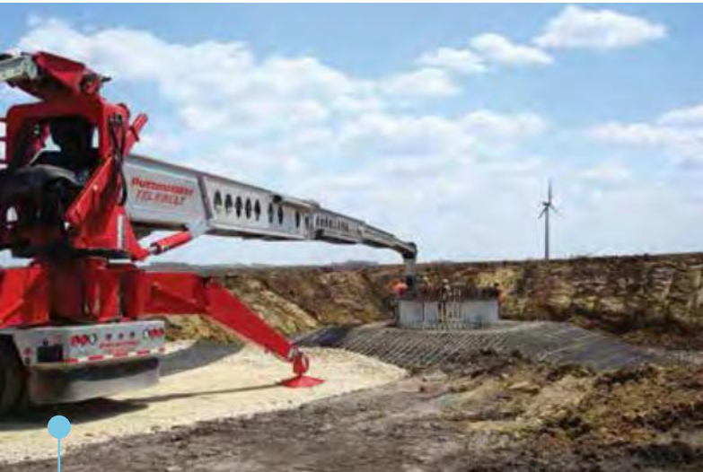
Telebelts can place concrete for the tower bases and roadbase material for site access roads at wind farm projects.
