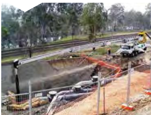
Placing unpumpable concrete
