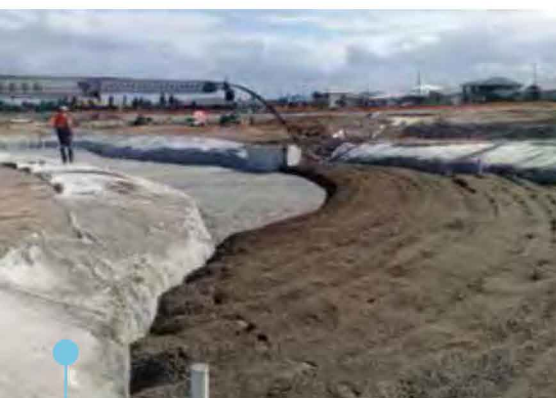
This Telebelt remained on site to place both materials over geotextile for this detention basin.
