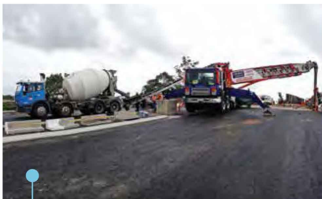
Pouring cast in situ barriers for a railway overpass. The reach of the Telebelt can generally avoid having trucks on the bridge, and minimises disruption to other works.
