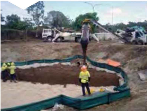
Backfilling over geotextile in a detention basin
