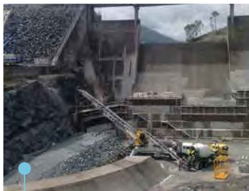
Placing concrete at a dam upgrade project. The ability to handle multiple materials and stiff concrete mixes is an asset on a remote site, compared to a pump.
