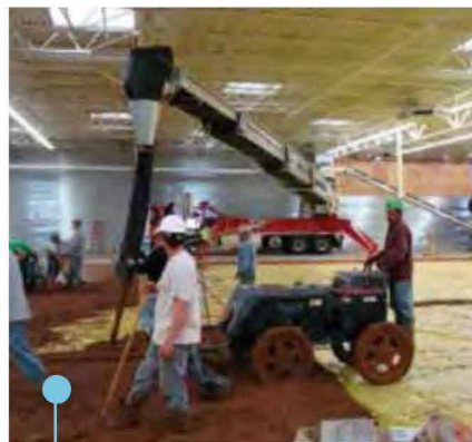
Placing concrete indoors for high productivity laser screeding equipment. A Telebelt is faster than a pump, handles stiff mixes and can work with lower head height.
