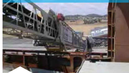
Radial stacking conveyors
