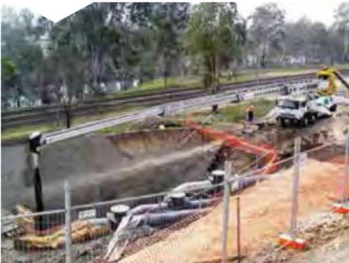
Placing unpumpable concrete
