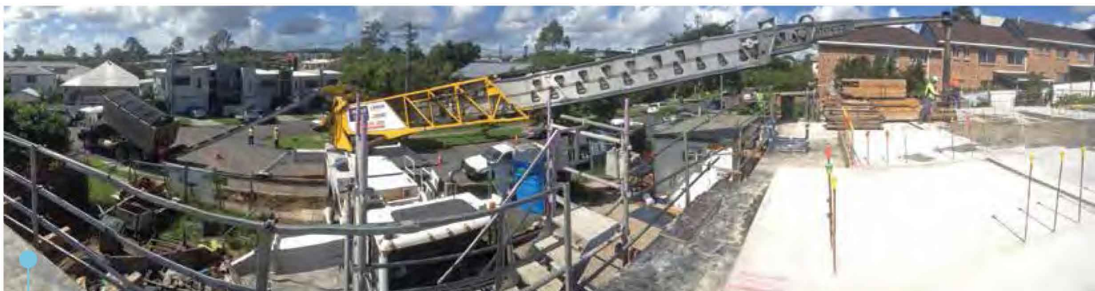
Panorama image of tipper on the street discharging directly into the feed belt hopper via a grain chute, with the telescopic placement belt used to place 20mm drainage gravel around a unit block slab at an elevated level.
