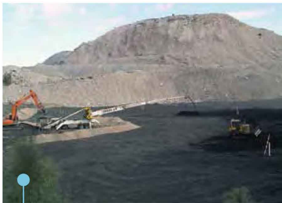
Capping a tailings dam by placing coal rejects over geotextile for a swamp dozer to push out.
