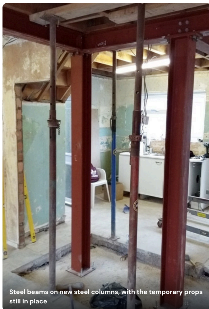
New beam installed and propped while it is packed and pinned up
