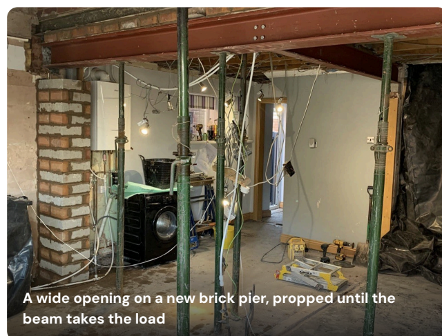
New beam installed and propped while it is packed and pinned up
