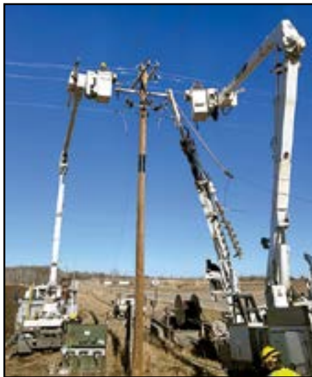
Wild Rice Electric Cooperative crews working on upgrading a feeder.
