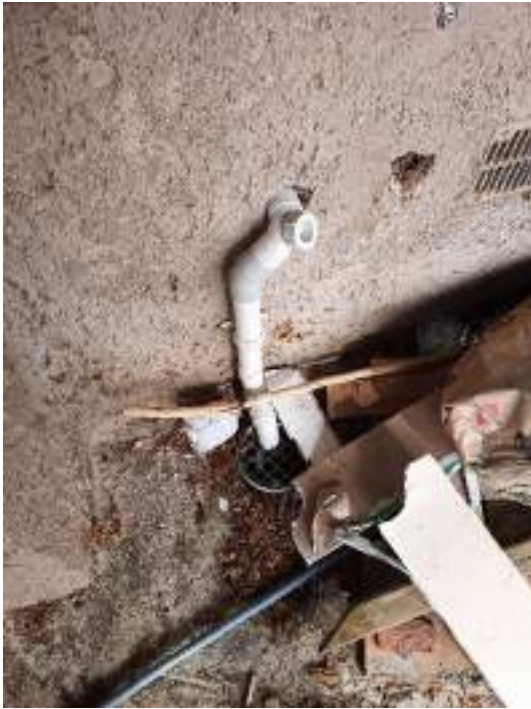
Waste pipe to the gully trap outside the ensuite
