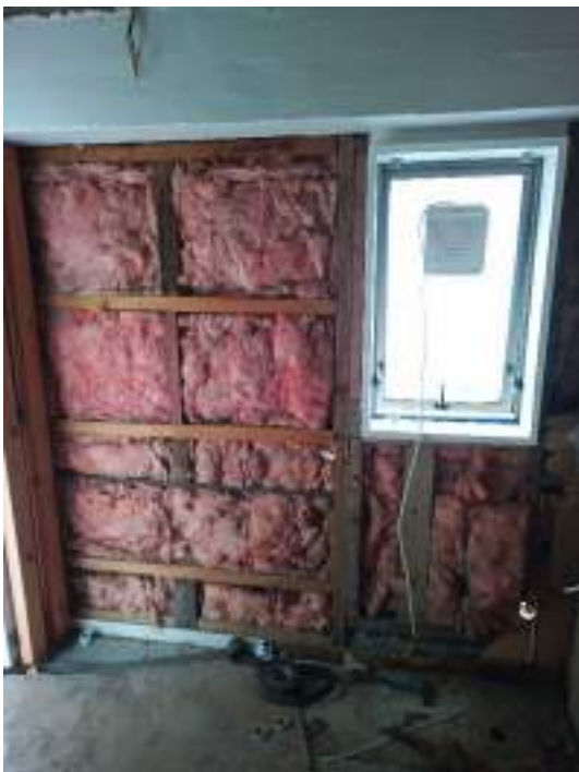
Insulation and original timber framing was visible to the external walls of the ensuite
