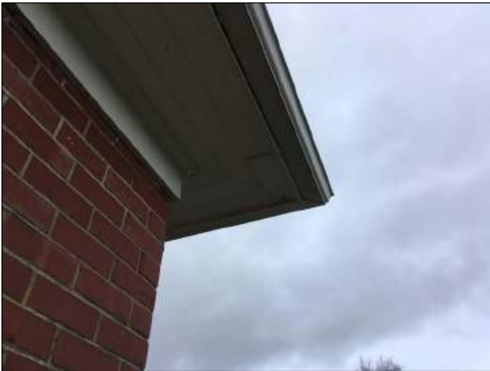
Plate 4: Patched up soffits
